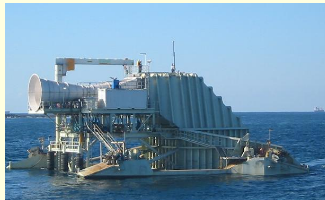
Oscillating Water Column
