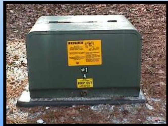
Padmount Transformer for Underground System
