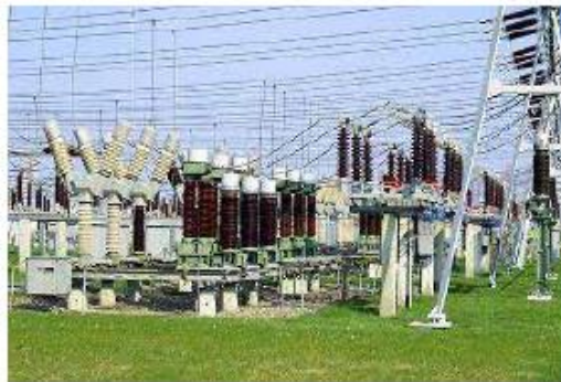
Circuit Breakers
