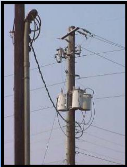
Overhead Transformer Bank & Service
