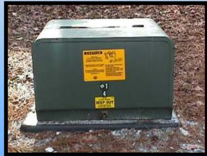
Padmount Transformer for Underground System
