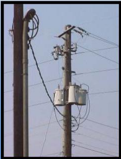
Overhead Transformer Bank & Service
