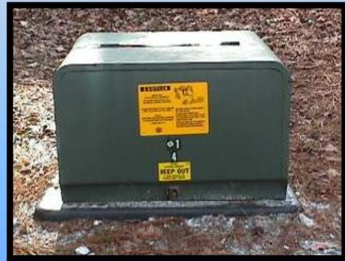
Padmount Transformer for Underground System
