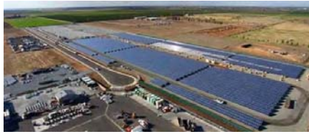
5 MW Fixed-Tilt Ground-Mount System near Porterville, CA
