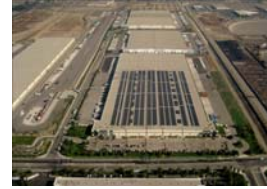
2 MW Warehouse Roof Mounted PV System near Fontana, CA
